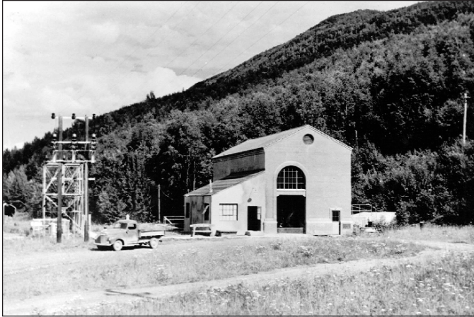
Figure 16. AL&P powerhouse as it appeared with lean-to addition added in 1935 and the relocated transformers to left. Courtesy of National Archives.
