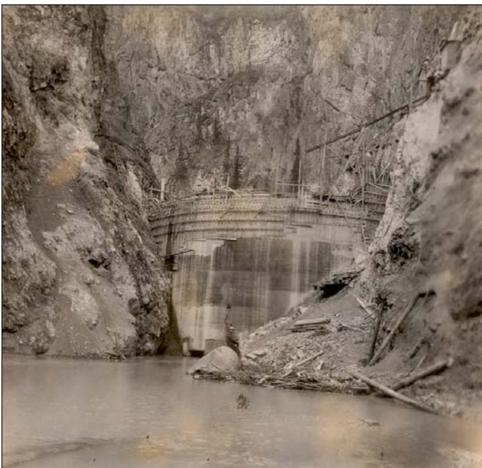
Figure 12. Upstream face of diversion dam under construction.
