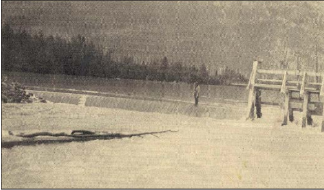
Figure 14. Eklutna Lake spillway, discharging 1,500 cubic feet of water per second. July 7, 1929.
