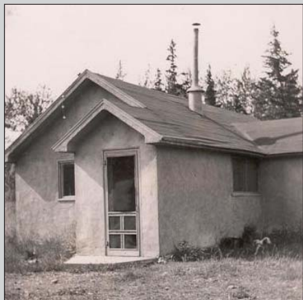
Figure 26. Frank M. and Maxine Reed's cottage at Eklutna. This building was used as an office until Frank M. was hired in 1937.
