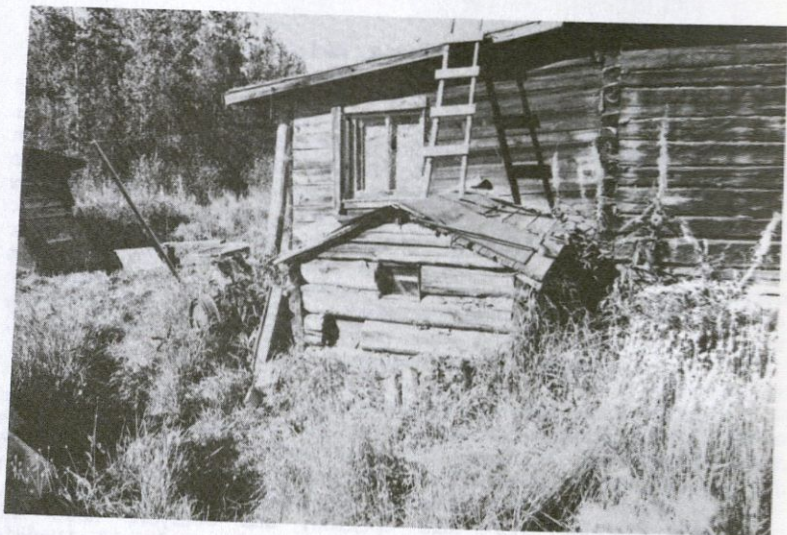
Home of Mike and Katherine Theodore at Eklutna, built in 1927 by Theodore. Steam bath (left) is attached to enclosed porch, so it can be entered from inside during cold months. Main house (right) and steam bath are of logs; porch is frame. Ladder makes repairing the tarpaper roof easier. (AFC, 1981)
