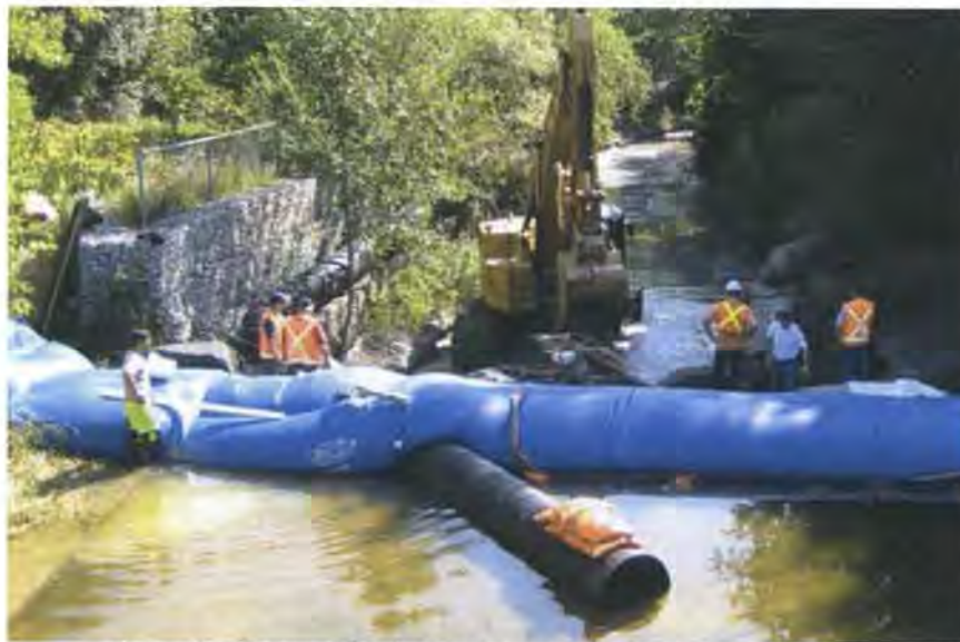
Figure 3. Photograph of a similar, water-inflated diversion dam courtesy of Hydrological Solutions, Inc.
