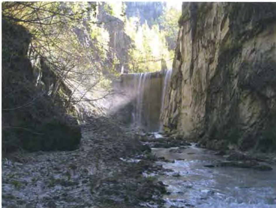
Figure 1. Photograph looking upstream at lower Eklutna River dam, May 2009 (USACE 2009).
