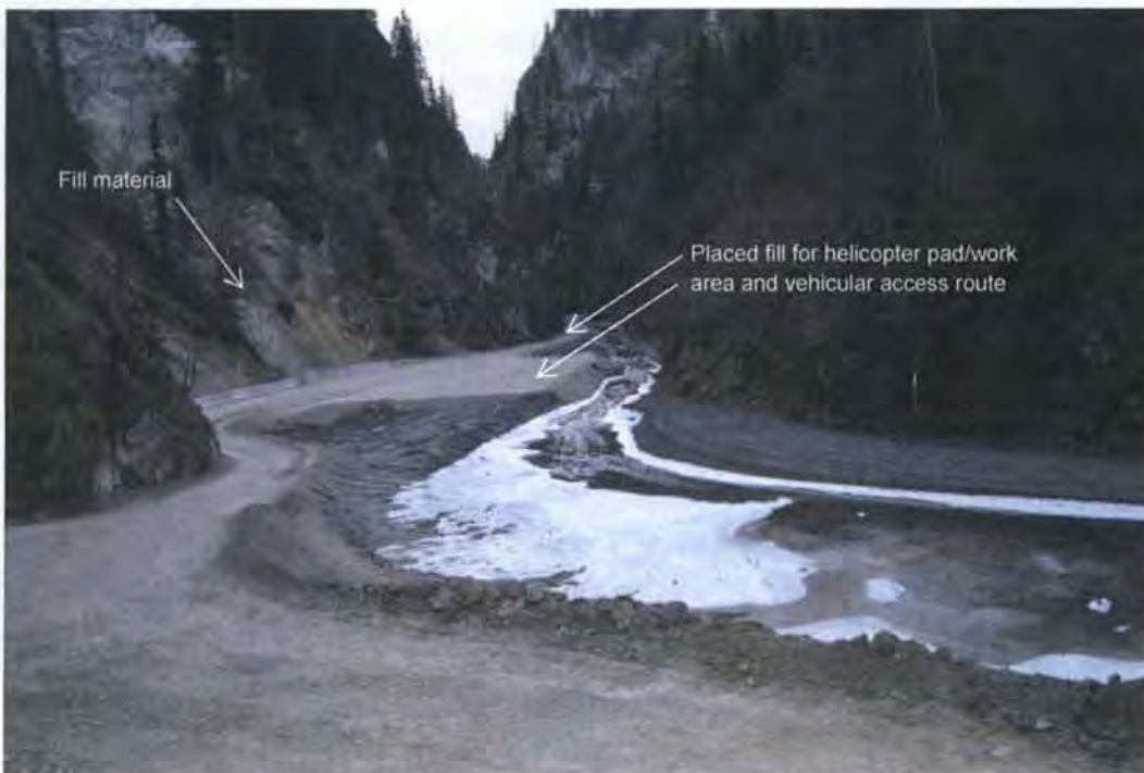
Figure 2. Looking upstream into canyon from lower staging area; fill placed in 2016 for the construction of an access route and helicopter landing pad/work area adjacent to the Eklutna River visible. Photo credit: Joe Miller, HDR, October 18, 2016.
