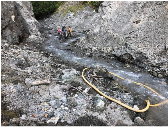
Figure 27: Plastic tubing construction debris
