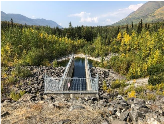
Figure 1: Spillway looking downstream
