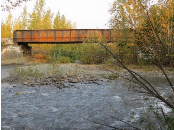
Figure 17: Looking downstream at the railroad bridge
