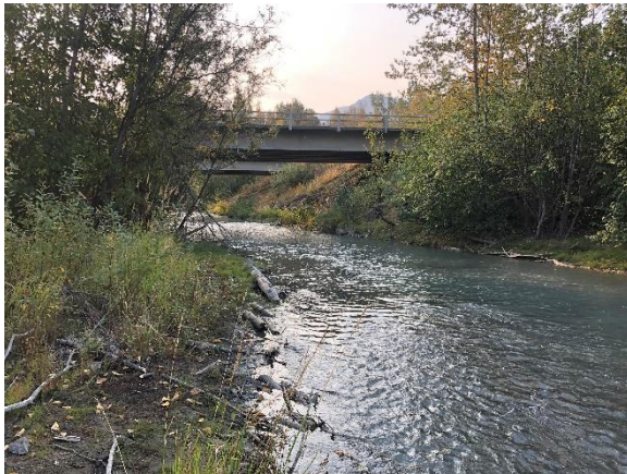
Figure 19: Looking upstream at Glenn Highway bridges
