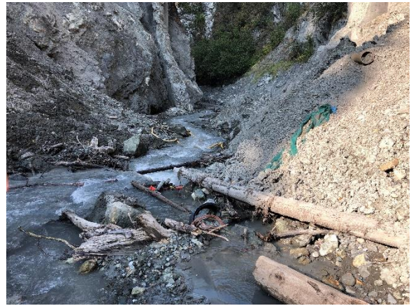
Figure 28: Miscellaneous construction debris
