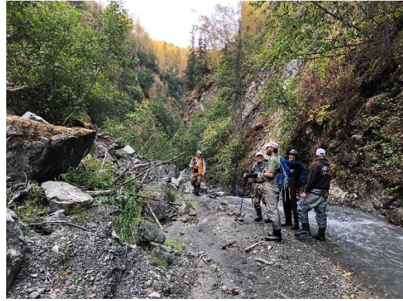
Figure 23: Channel constriction from landslide
