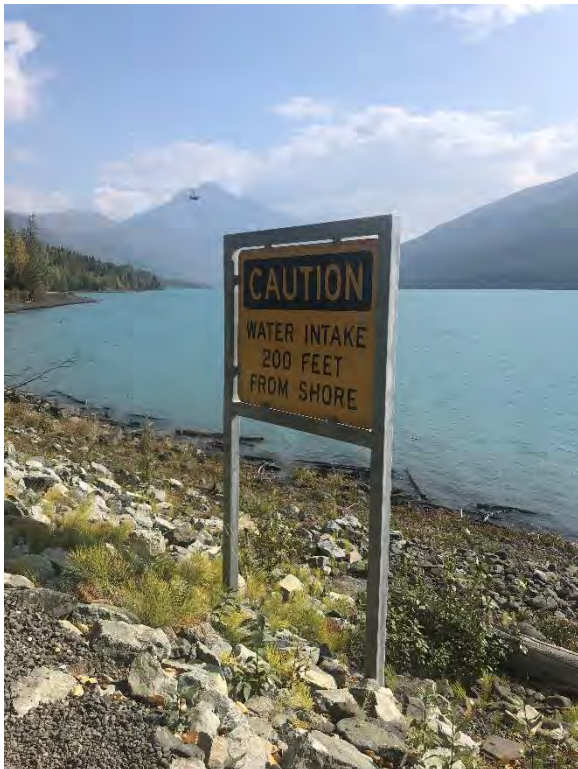
Figure 4: Power tunnel intake
