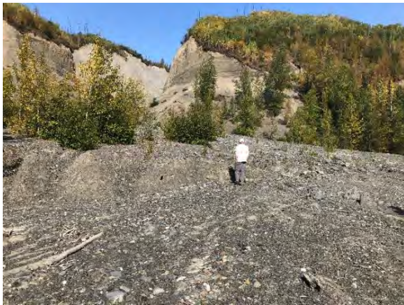
Figure 15: Large active landslide area
