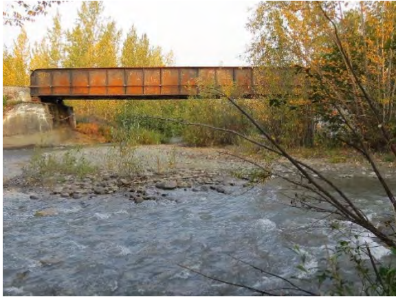
Figure 17: Looking downstream at the railroad bridge
