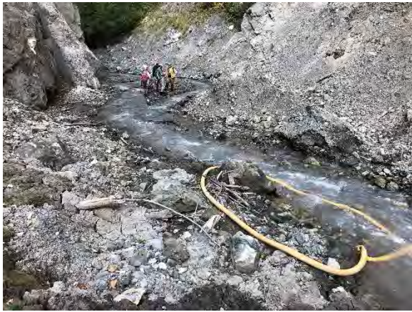
Figure 27: Plastic tubing construction debris
