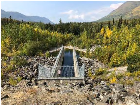
Figure 1: Spillway looking downstream
