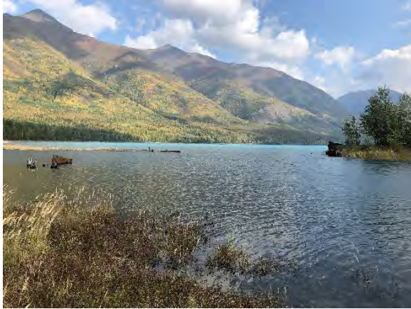
Figure 3: Remnants of old dam structures at lake outlet
