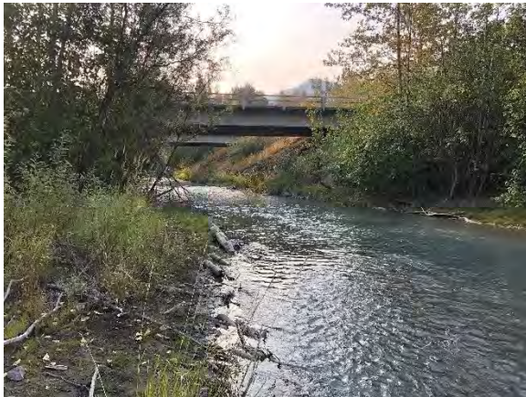
Figure 19: Looking upstream at Glenn Highway bridges
