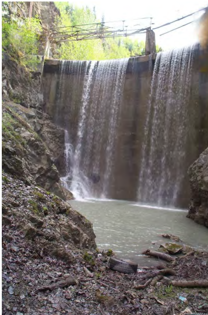
Photo 1: Backfilled Lower Eklutna Dam
