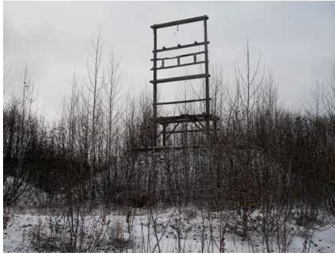
Figure 6. The remains of an electrical substation perched above existing ground level after approximately 20 vertical feet of aggregate was removed by mining operations.
