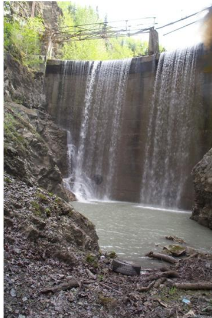
Figure 5. Backfilled Lower Eklutna Dam
