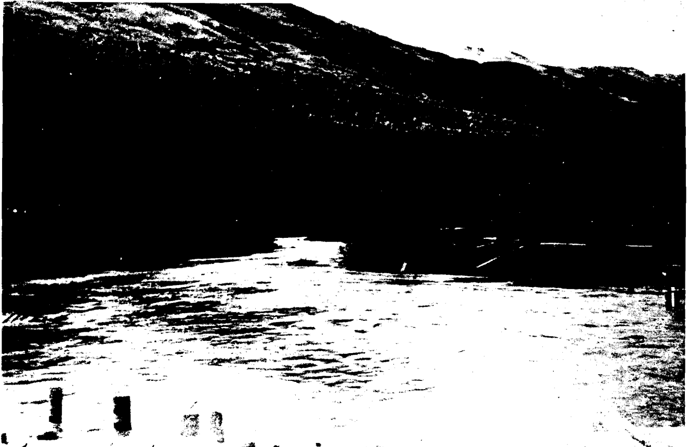
RIVER CHANNEL BELOW GATES (BELOW)
