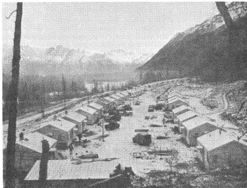
Figure 102. --Temporary and permanent houses under construction at Eklutna Government camp. P783-908-459. November 27, 1951.
