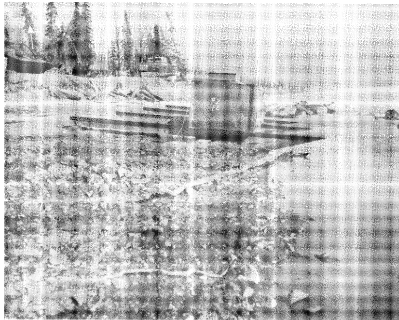
Figure 104. --View of assembly area for dredge at Eklutna Lake showing one steel pontoon and steel skids on which assembled dredge will slide into lake. P783-908-788, May 2, 1952.
