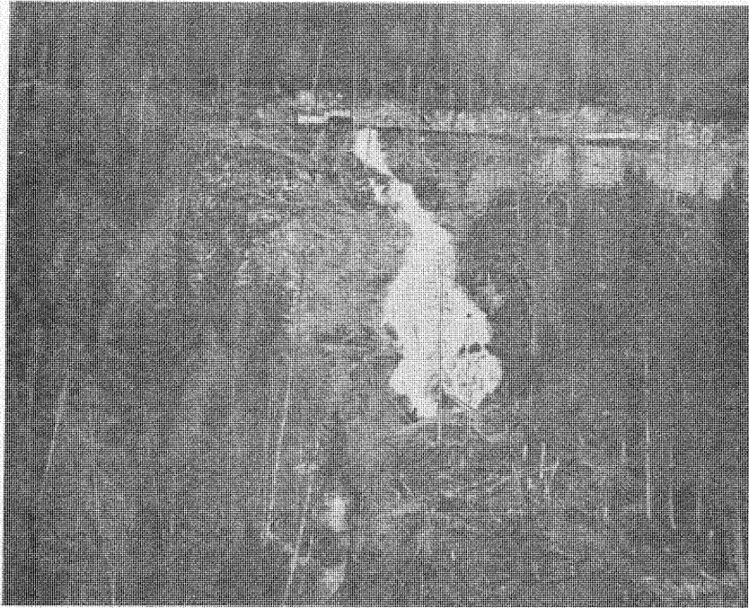
Figure 111. --Tunnel drainage from fault at station 208+70, cascading down slope toward highway. Flow was estimated at 7,800 gallons per minute. P783-908-1153, November 10, 1952.
