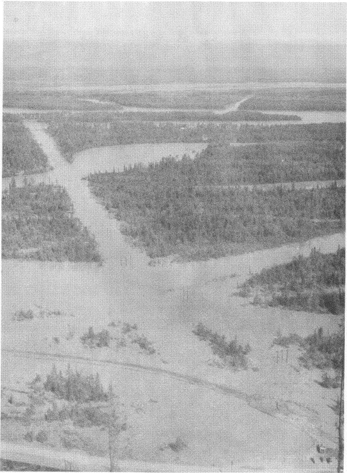
Figure 16. --General view from tunnel adit portal showing conditions at height of Knik River flood during the Lake George breakup. Note powerplant and tailrace embankment in foreground. P783-908-1665, July 26, 1954.
