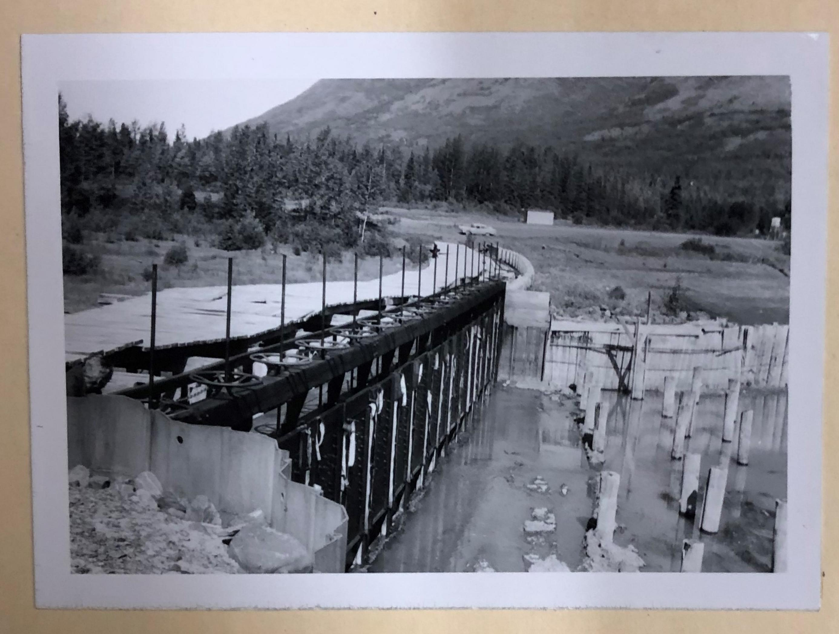
P783-906-2358 Eklutna Powerplant - Alaska. View of the dam and spillway gate structure at Eklutna Lake. This structure, built by private interests in 1929, was declared unsafe for impounding water after the March 27 earthquake. All gates were locked open throughout the spring run-off and plans were started immediately by the Bureau of Reclamation for the construction of a new spillway and gate structure.
