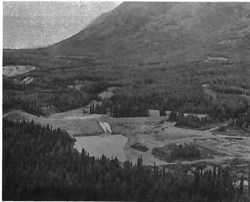
Figure 56. View of completed Eklutna Dam, showing the upstream face and the spillway inlet. P783-D-58572, August 1967.
