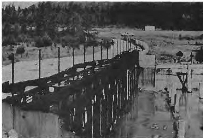
Figure 21. --View of spillway gate structure of existing dam. P783-906-2358NA.
