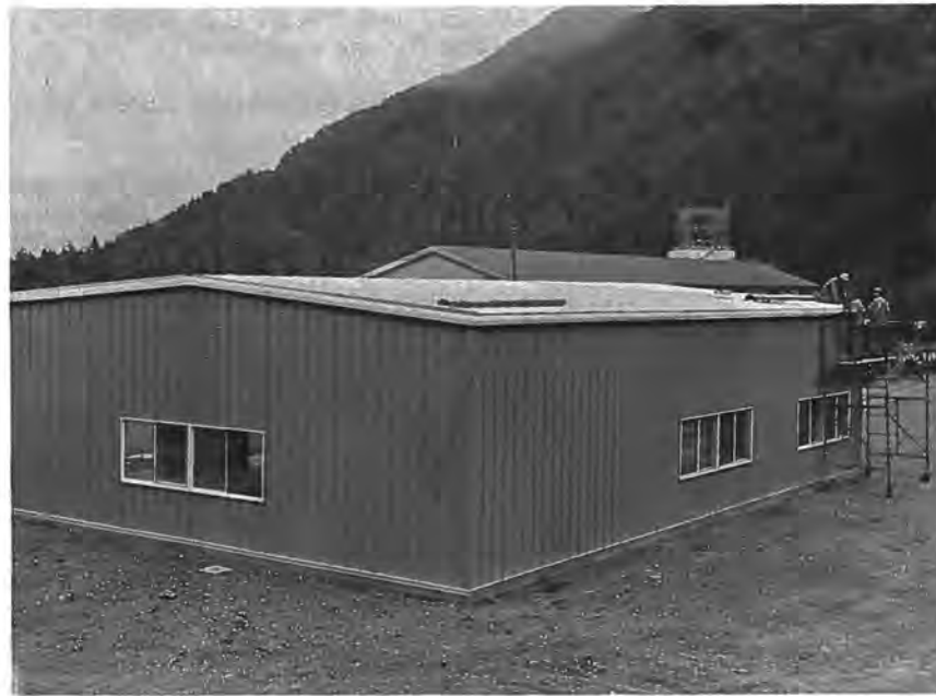
Figure 31. --New automotive repair shop. P783-908 C&R-192A, September 3, 1965.
