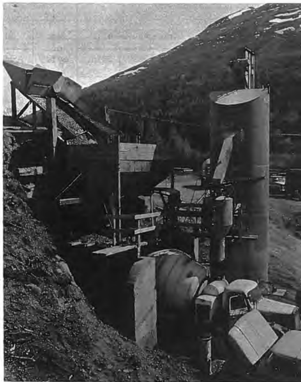
Figure 64. --Contractor's batching plant located at the damsite. P783-908 C&R-130A, June 16, 1965.
