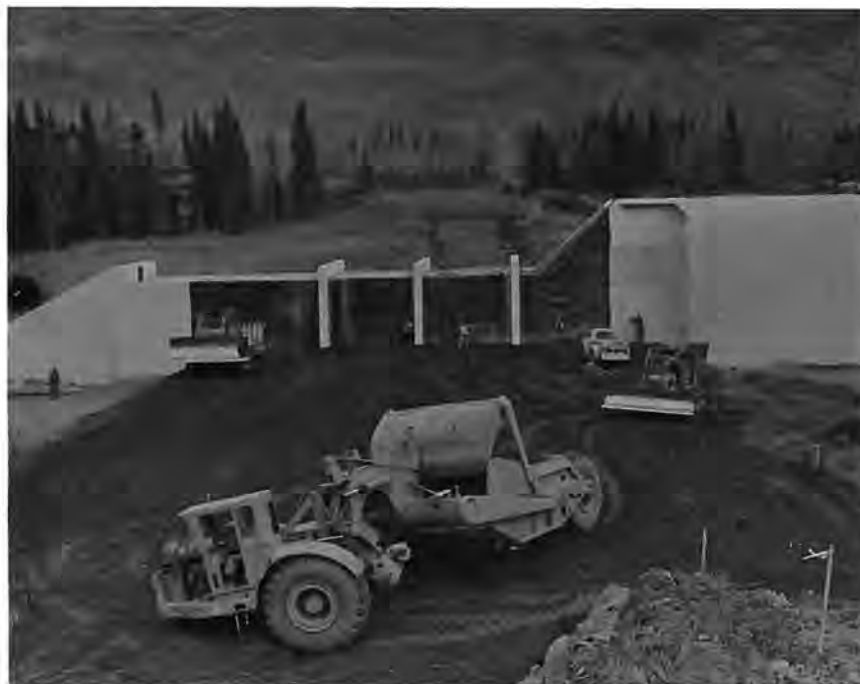
Figure 59. --Placement of zone 1 embankment on the dam. P783-908 C&R-194A, September 14, 1965.
