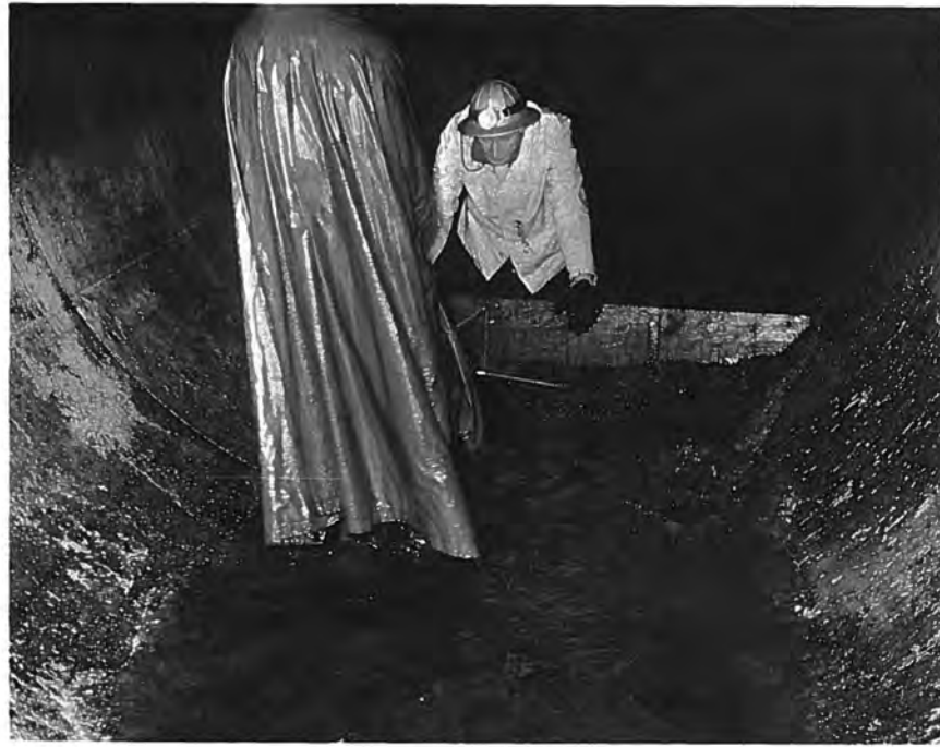
Figure 41. --View of tunnel mucking operation by Bureau force-account employees. Sand and rock is being moved toward the adit tunnel by means of a movable plywood dam utilizing the head developed by the leakage water to assist motivation. P783-906-2326, May 1964.
