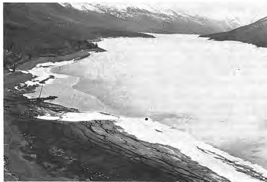
Figure 14. --View of shoreline of Eklutna Lake in the vicinity of the intake structure after the earthquake. Intake structure is located at left center of photograph on shoreline. P783-D-44348-A.
