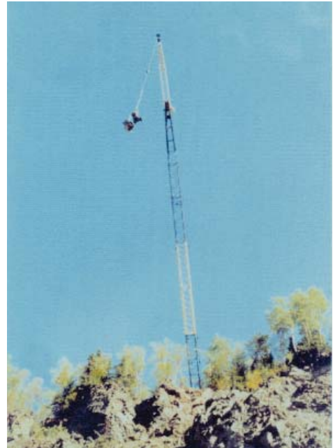
200' crane boom hoisting atop 300' Eklutna River Canyon cliff.
