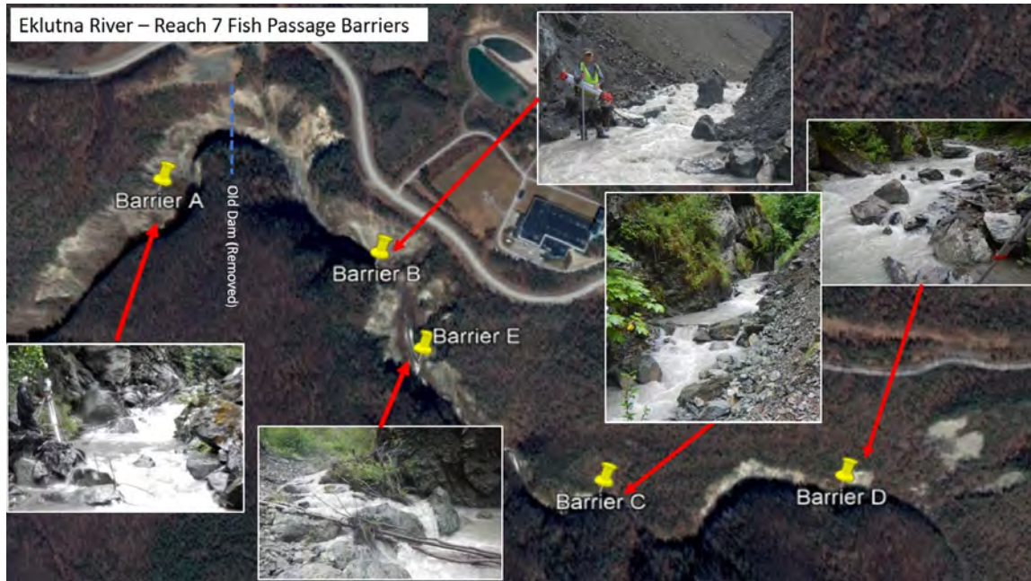
Figure 3-1 Locations of potential barriers within Reach 7 of the Eklutna River surveyed for passage analysis. Sites A – D were identified during 2021 surveys; Site E was added during the 2022 survey.
