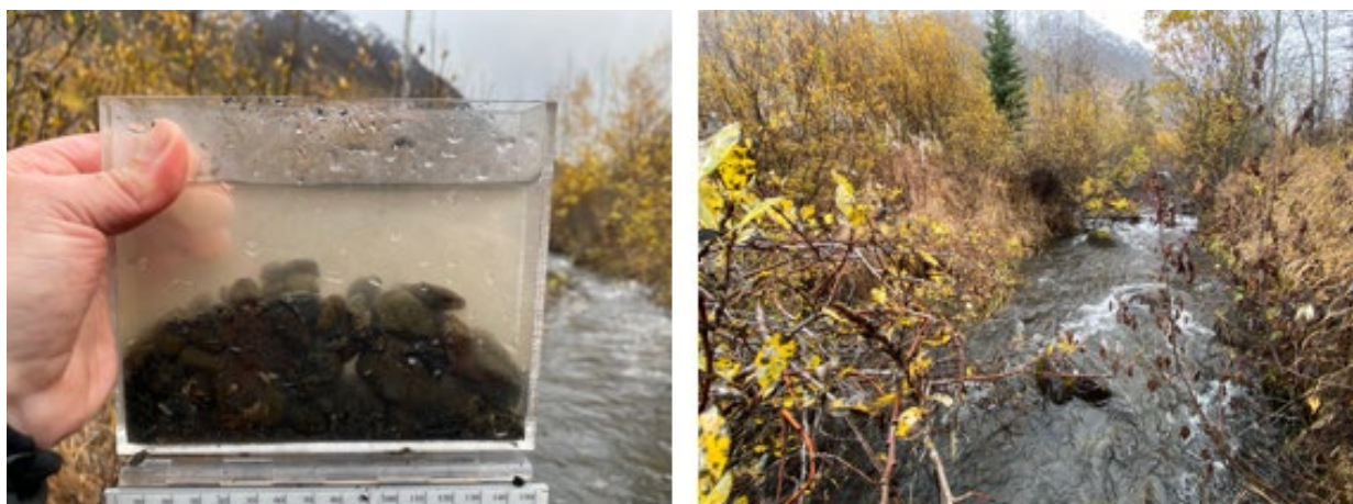
Figure 1-6 Tributary 4 downstream of the culverts under the Eklutna Lakeside Trail (right) and example of substrate size in limited areas with gravel (left).
