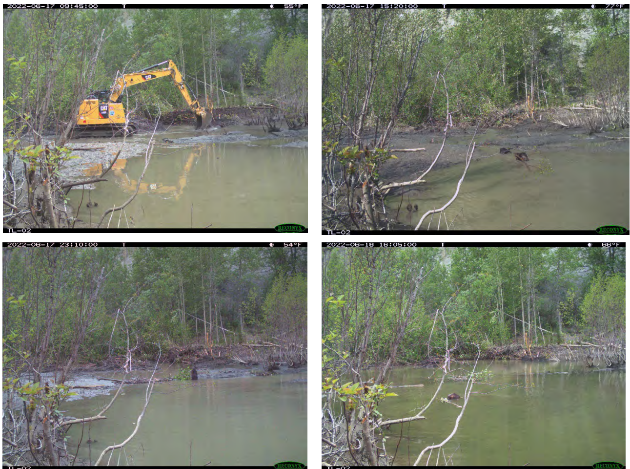
Figure A.3-16. Photograph series documenting the mechanical breaching of a beaver dam and the nearly complete repair by the following day.
