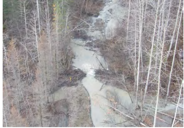
Figure A.2-6. Inactive Dam-05 in the middle Eklutna River drainage just upstream of the canyon and near the lower AWWU access road.
