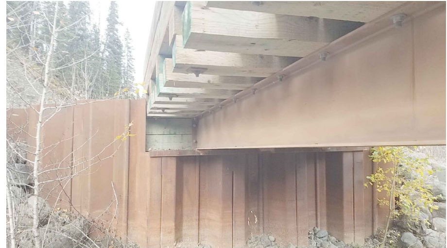
PROPOSED CROSSING BRIDGE EXAMPLE - LOOKING AT RIVER-LEFT ABUTMENT FROM RIVERBED SCALE: NTS
