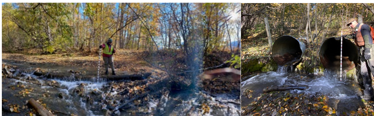
Figure 3.1-6. Lach Q’atnu Creek transition from varial zone to low-gradient stream (left) and paired culverts 250 meters from the location lake. Photos from September 30, 2021.
