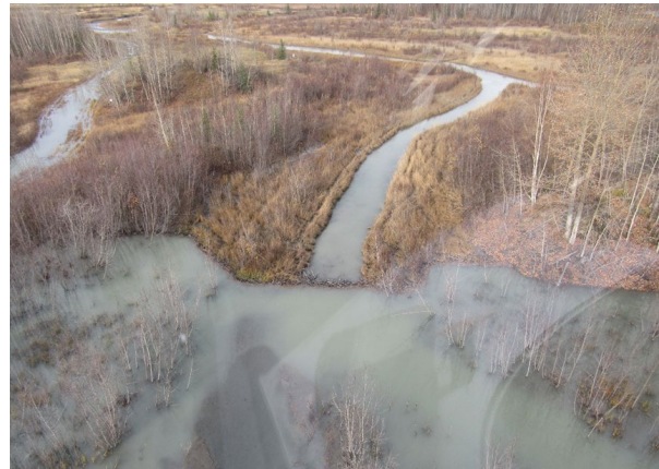
Figure A.2-4. Active Dam-03 in the lower Eklutna River area (middle). Dam-04 is just off-photo to the right.
