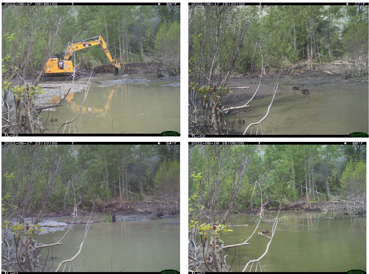
Figure A.3-16. Photograph series documenting the mechanical breaching of a beaver dam and the nearly complete repair by the following day.
