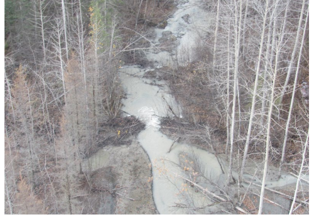
Figure A.2-6. Inactive Dam-05 in the middle Eklutna River drainage just upstream of the canyon and near the lower AWWU access road.
