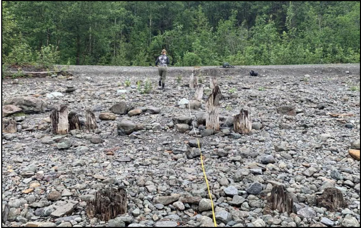
Figure 5.2-19. View to the north showing the pier arrangement and Eklutna Lakeside Trail in background.
