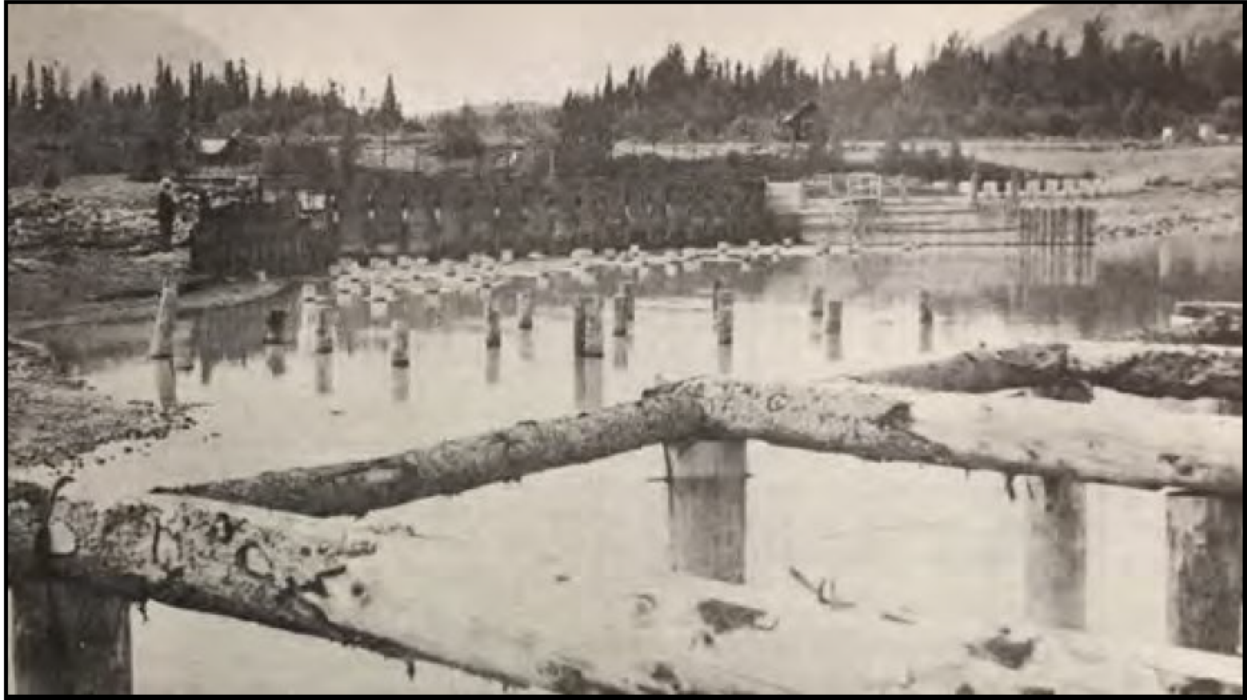
Figure 5.2-15. Cribbed log pier structure of the “breakwater weir” (bottom of frame) that restricted debris from entering the gate and spillway. Footings of this structure occur today as Feature 1. Photo from USBR (1948).
