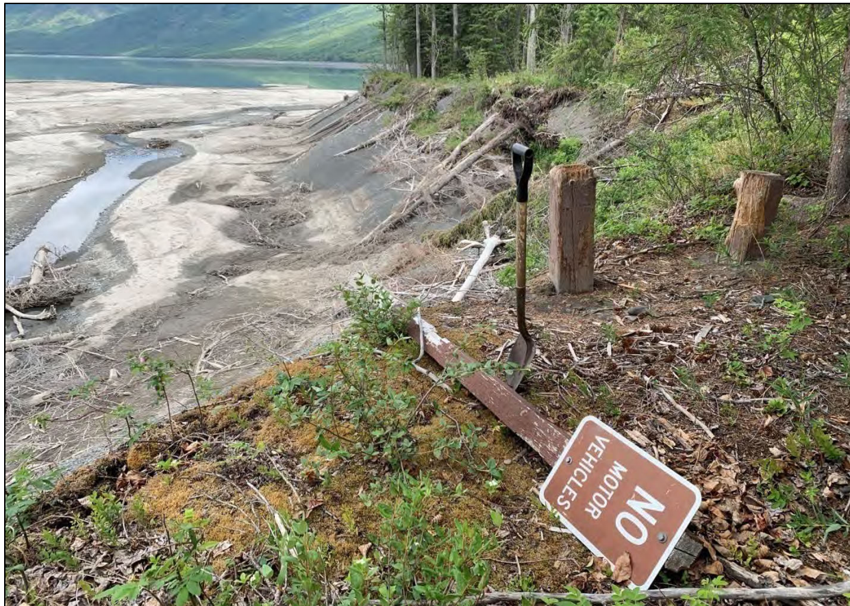
Figure 5.2-30. Eroded Chugach State Park trail just south of the former Eklutna Alex Cabin site. View to the northwest.
