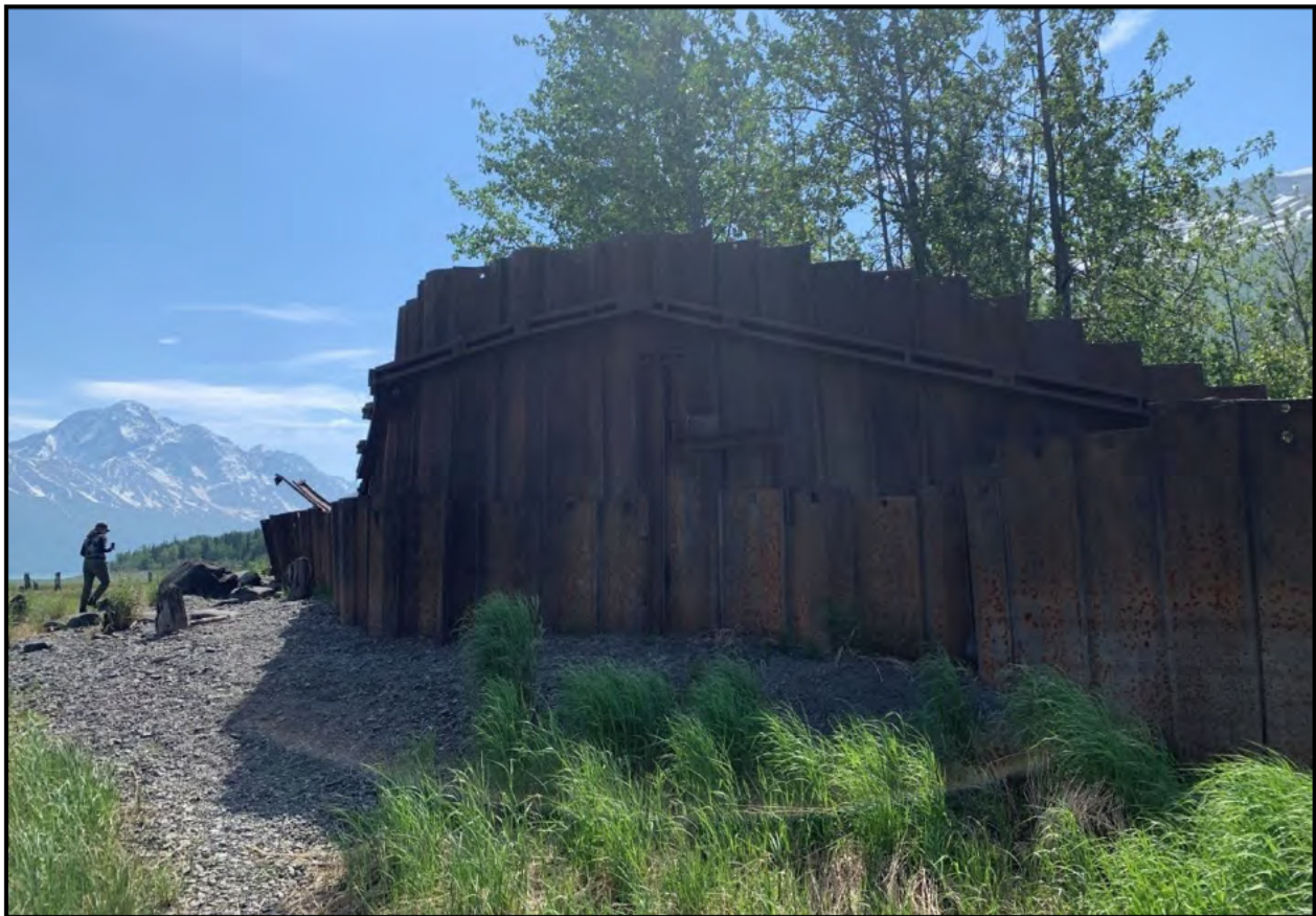
Figure 5.2-5. Feature 2 dam abutment on southern bank of the Eklutna Lake outlet. View to the southeast.
