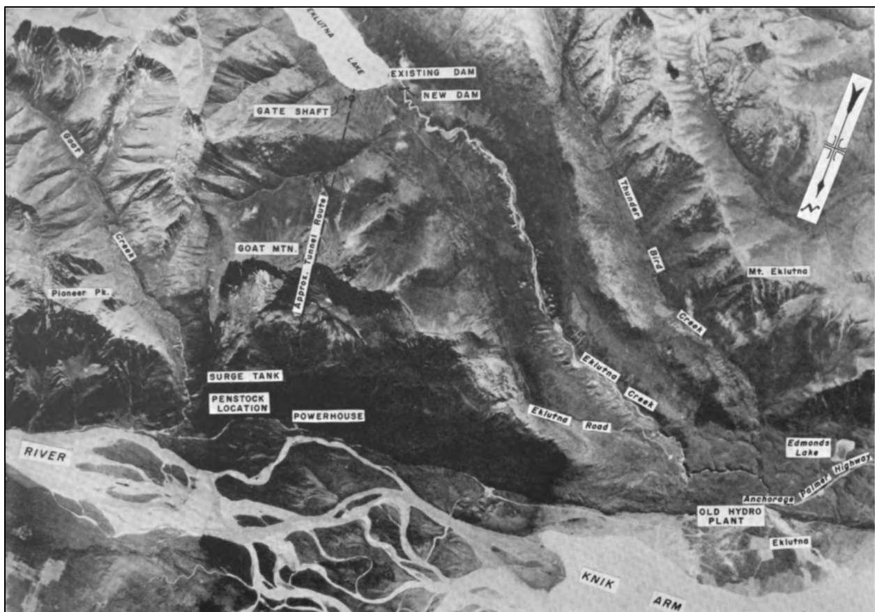
Figure 2.2-3. Aerial photo of Eklutna Project in 1967 (USBR 1967).
