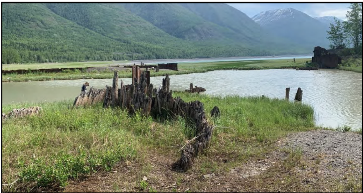
Figure 5.2-10. Feature 3, a partial dam abutment (foreground), showing its spatial relationship to Feature 2 across the man-made pond. View to the northeast.
