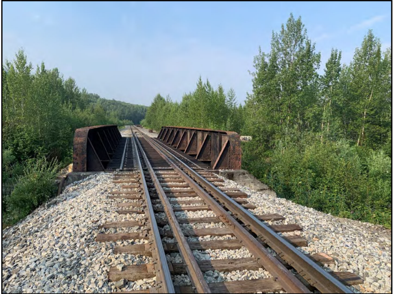
Figure 5.4-2. View to the west of the Eklutna River Railroad Bridge.
