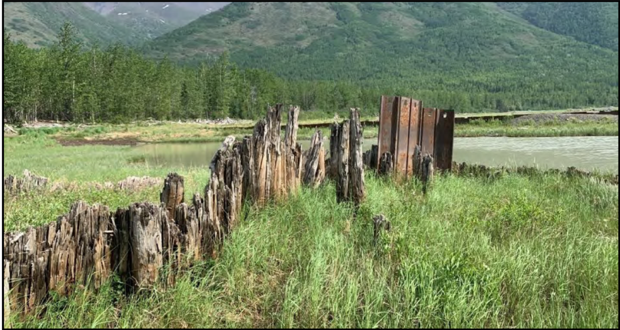
Figure 5.2-9. Feature 3, a partial dam abutment at outlet of Eklutna Lake. View to the north.
