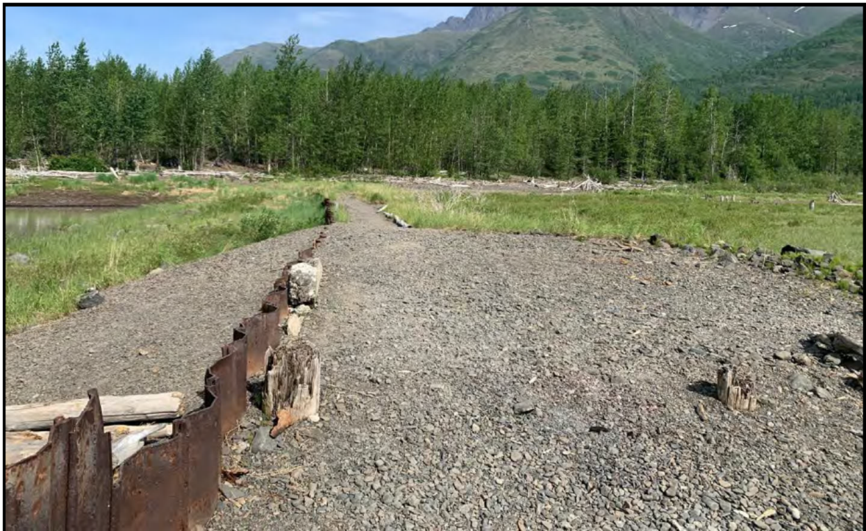
Figure 5.2-7. Feature 2 sheet pile and concrete-lined alignment on north side of Eklutna Lake outlet. This is currently used as a Chugach State Park foot path. View looking northwest.
