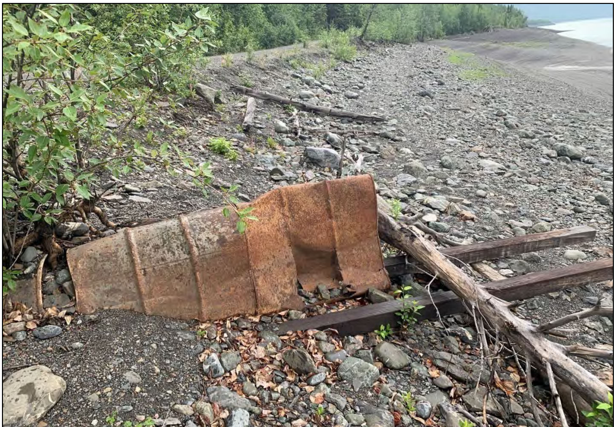
Figure 5.2-25. Culvert built of 55-gallon drums and wooden stringers. View to the east with the Eklutna Lakeside Trail to the left.
