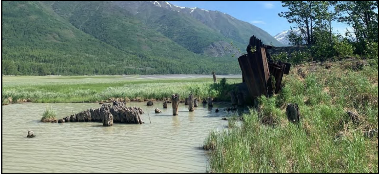
Figure 5.2-8. Feature 2 abutment with an irregular cluster of piers and planks in the center of the lake outlet. View to the northeast.
