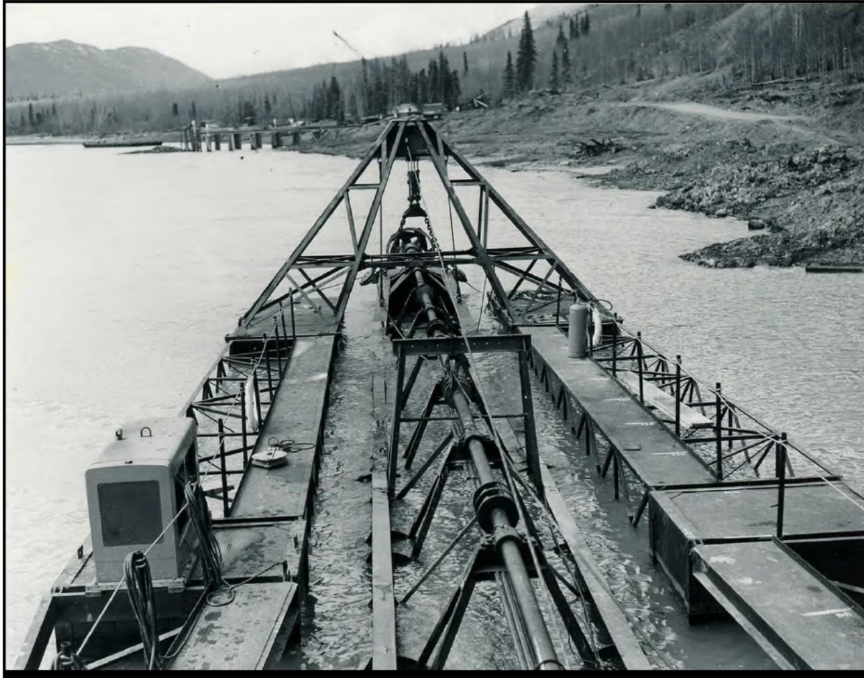
Figure 5.2-22. View of the temporary dock or wharf (background on shore) used during construction of the Eklutna intake tunnel.
