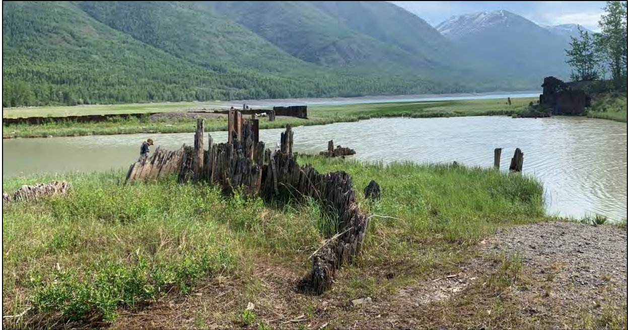
Figure 5.2-10. Feature 3, a partial dam abutment (foreground), showing its spatial relationship to Feature 2 across the man-made pond. View to the northeast.
