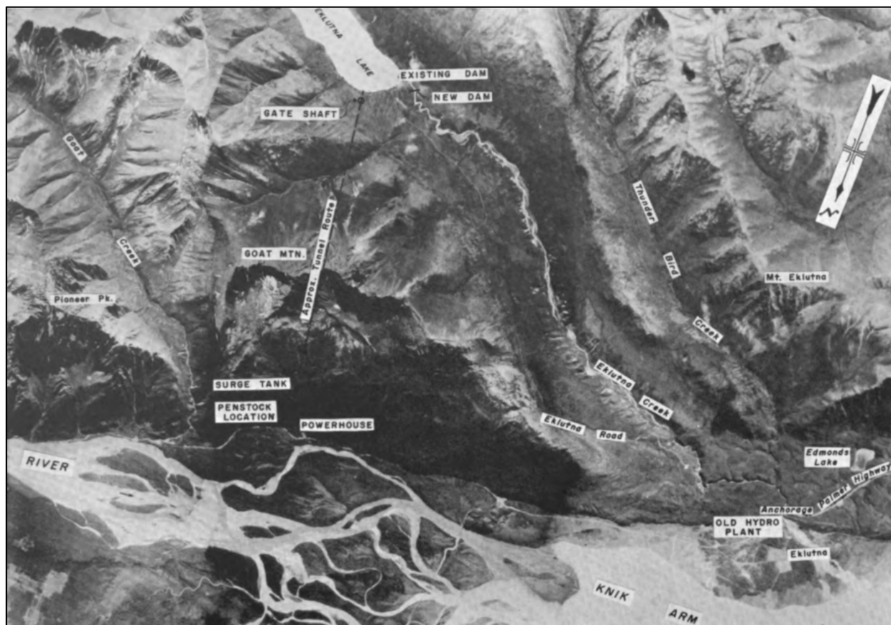
Figure 2.2-3. Aerial photo of Eklutna Project in 1967 (USBR 1967).
