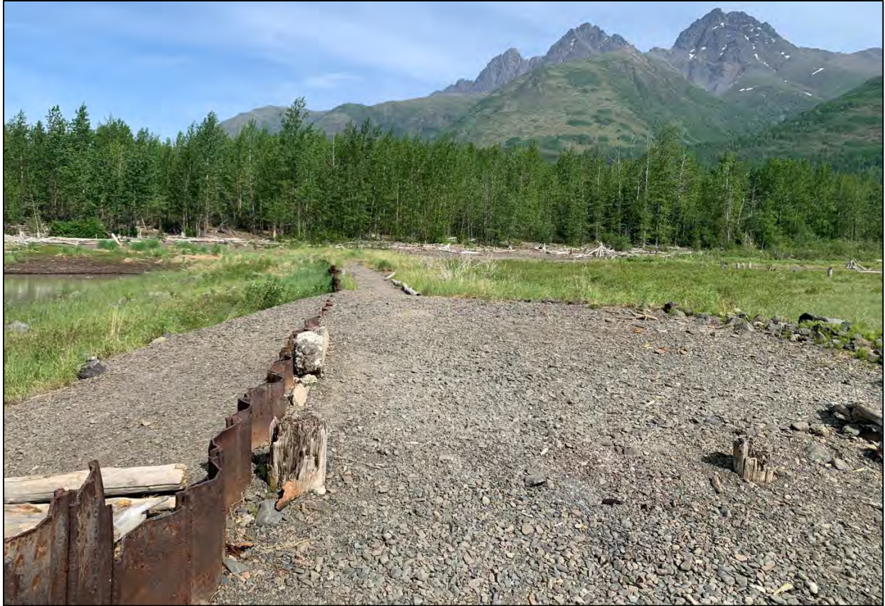
Figure 5.2-7. Feature 2 sheet pile and concrete-lined alignment on north side of Eklutna Lake outlet. This is currently used as a Chugach State Park foot path. View looking northwest.
