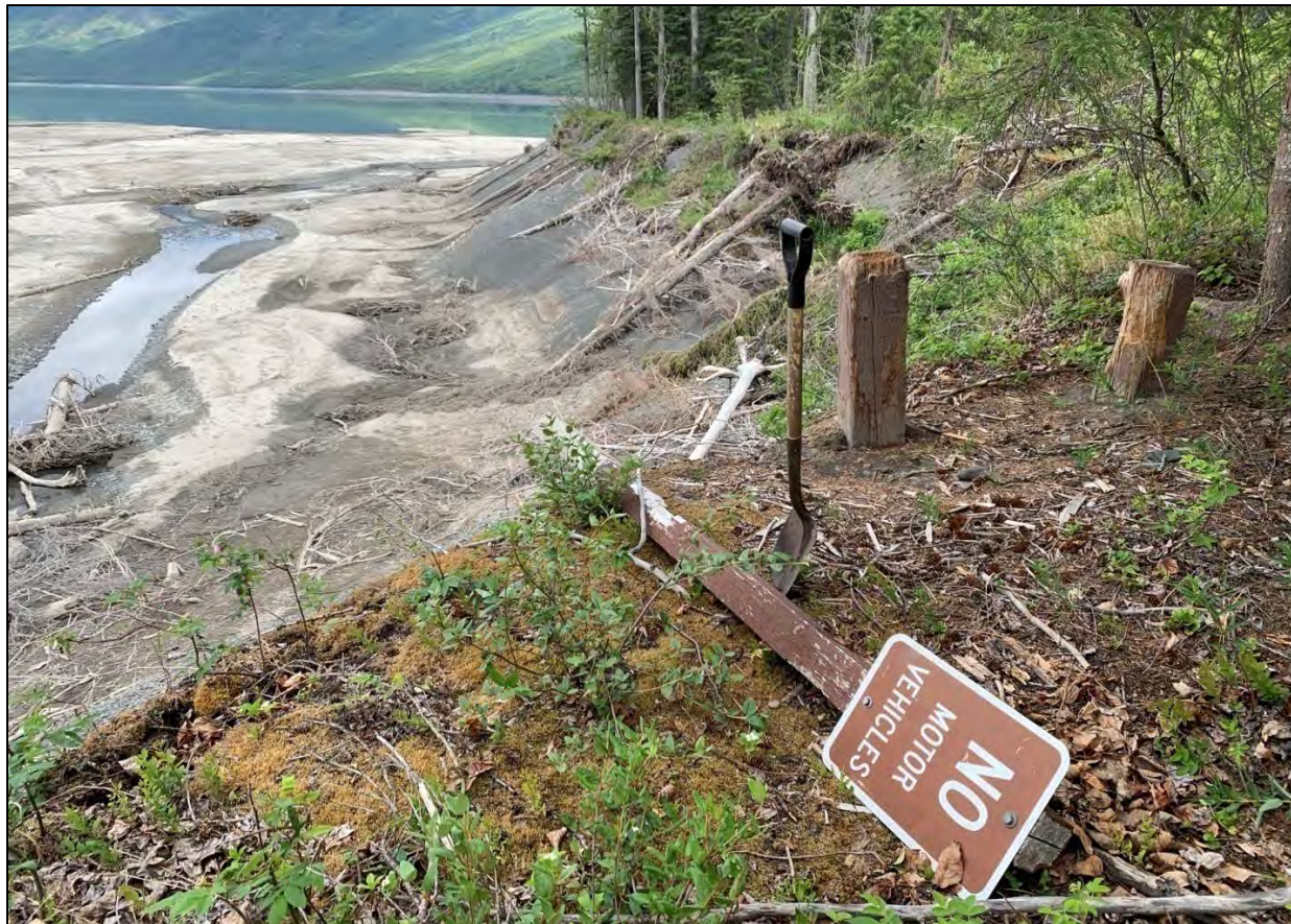
Figure 5.2-30. Eroded Chugach State Park trail just south of the former Eklutna Alex Cabin site. View to the northwest.
