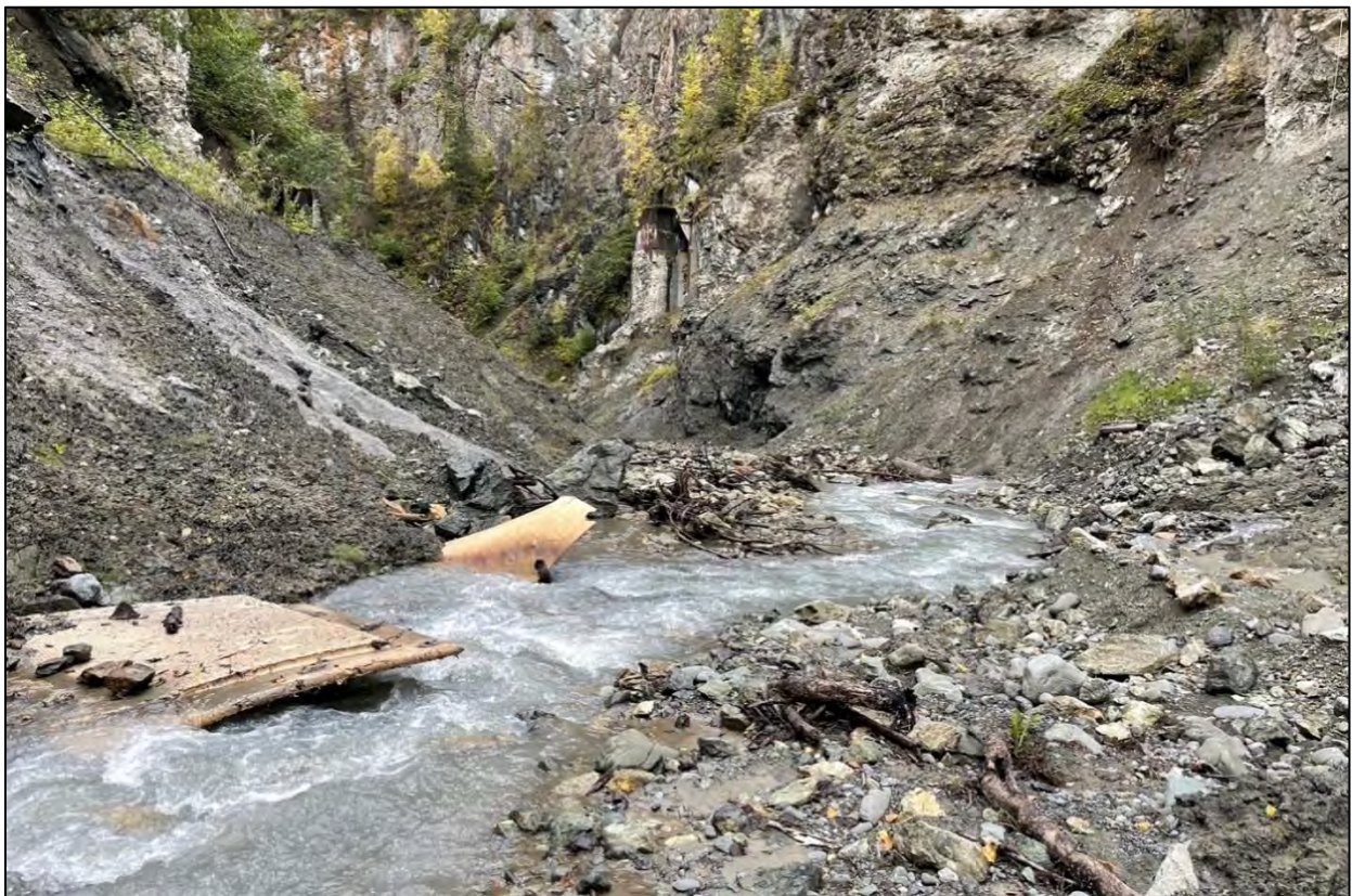
Figure 5.3-4. Debris upstream from the old dam site.
