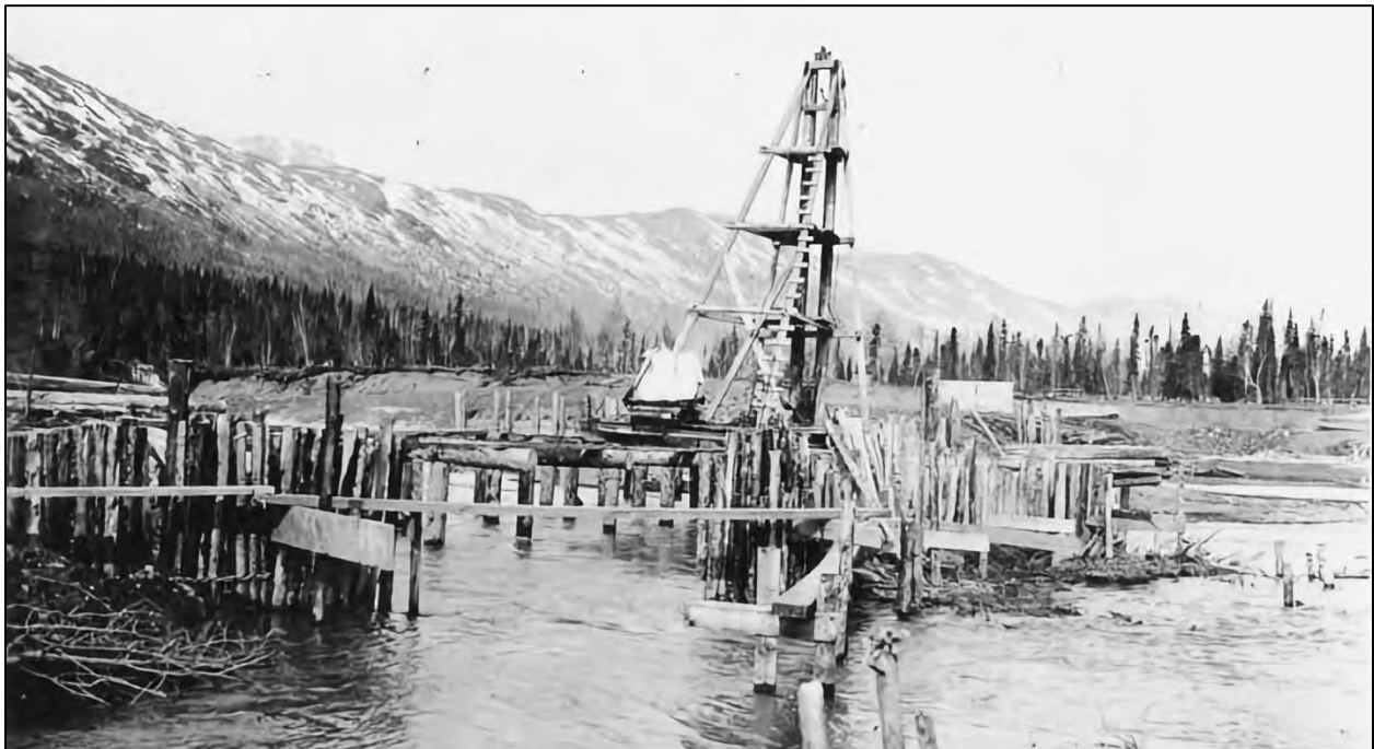
Figure 2.2-2. “Storage Dam at Outlet of Eklutna Lake” 1930–1932. (Walter W. Hodge Papers, University of Alaska Fairbanks, UAF-2003-63-67).
