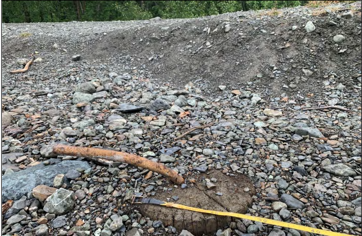
Figure 5.2-20. One of two log piers with threaded bolts. View to the northwest at the base of the Eklutna Lakeside Trail.
