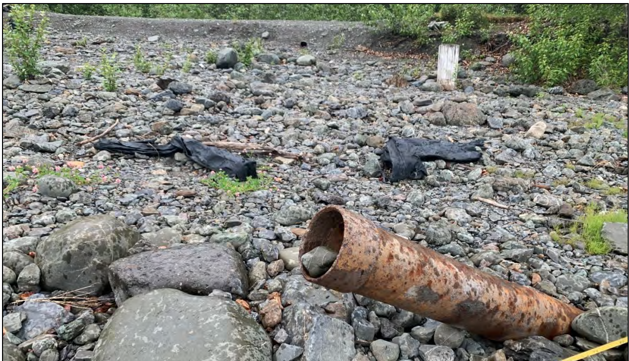
Figure 5.2-21. One of two threaded iron pipes within the pier arrangement. View looking north with Eklutna Lakeside Trail in background.
