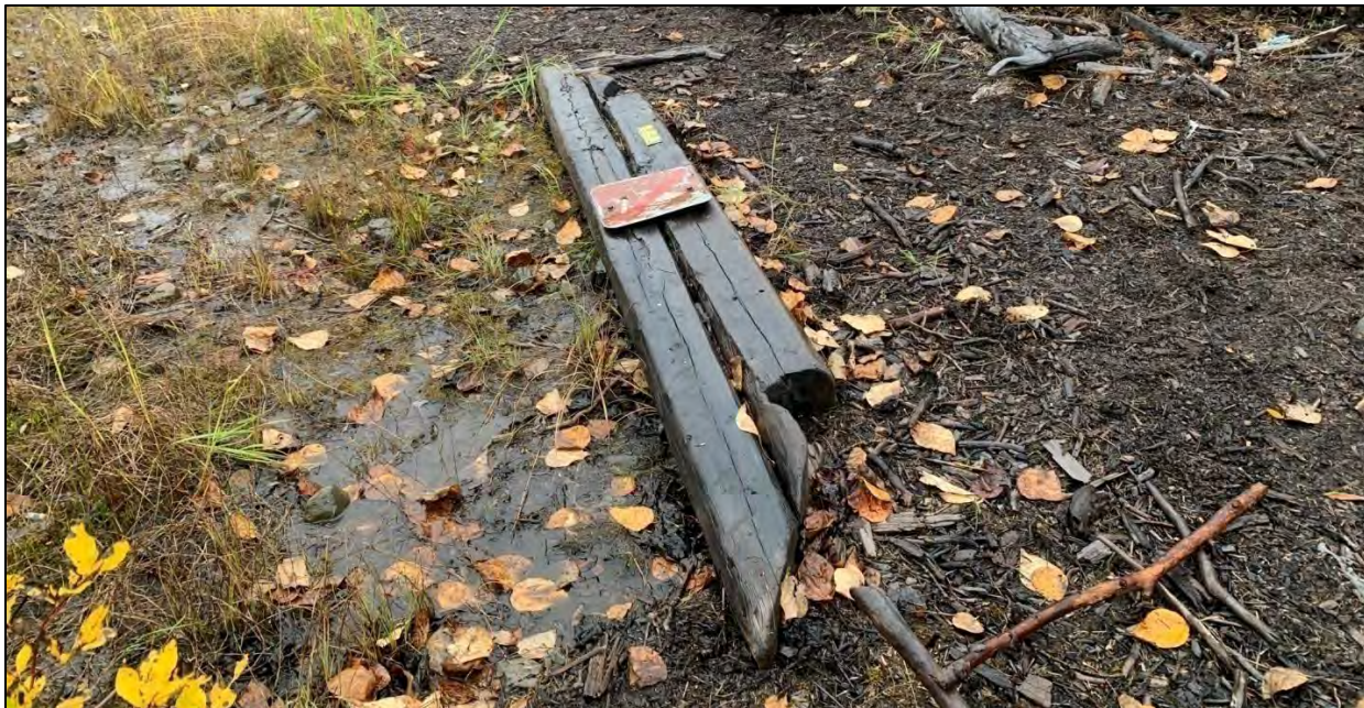
Figure 5.2-32. Two log courses of the displaced Eklutna Alex Cabin on the shore of Eklutna Lake, just north of its outlet.
