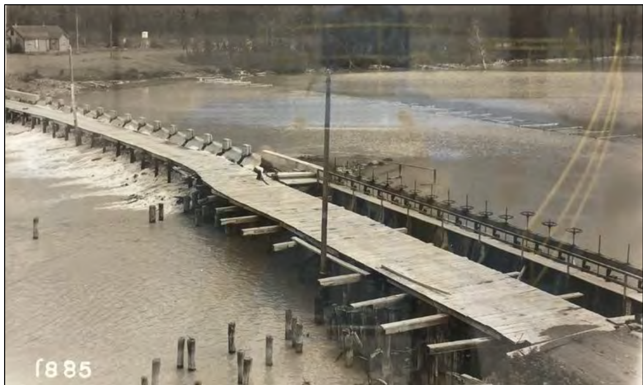
Figure 5.2-14. View of the Eklutna Dam in the early 1940s showing the dam and plank walkway in foreground (Feature 2). The separate “breakwater weir” cribbed alignment (Feature 1) is located to the right.
