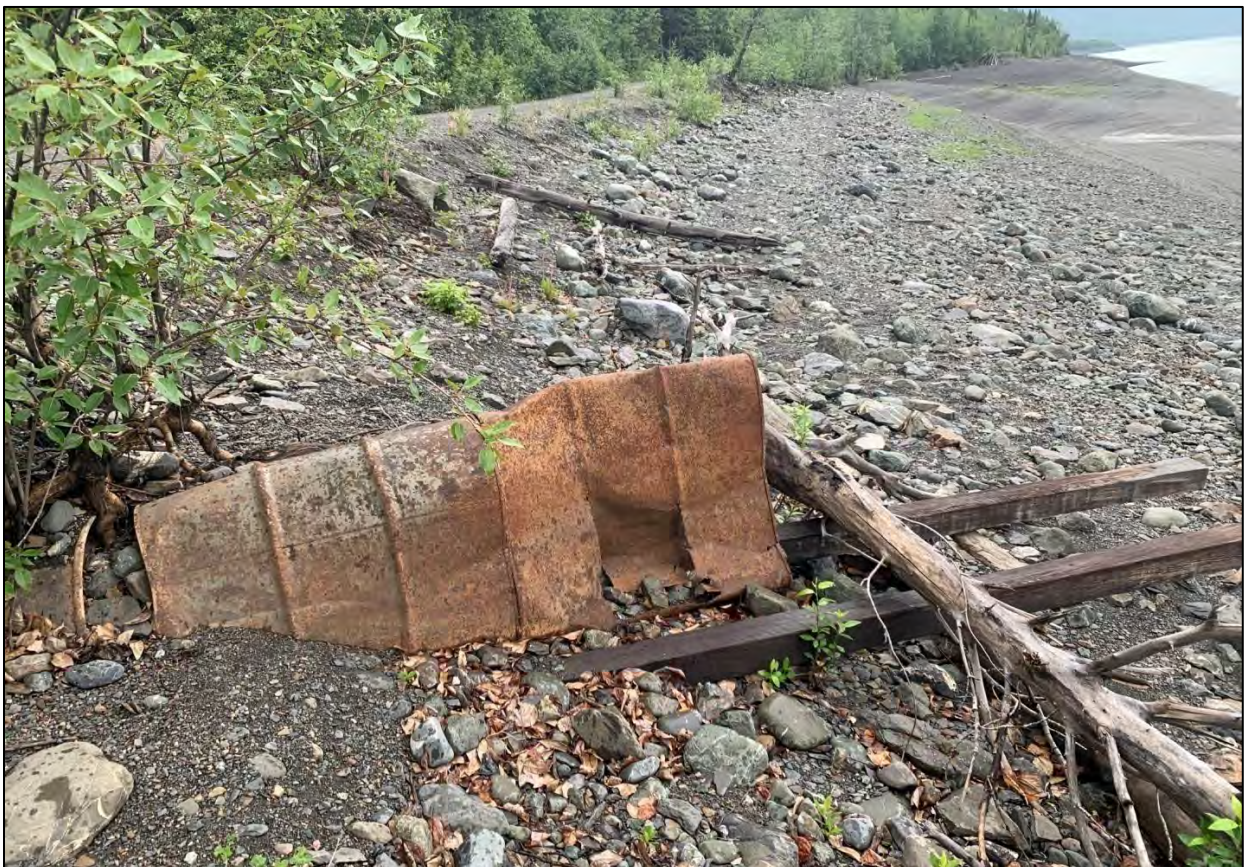
Figure 5.2-25. Culvert built of 55-gallon drums and wooden stringers. View to the east with the Eklutna Lakeside Trail to the left.
