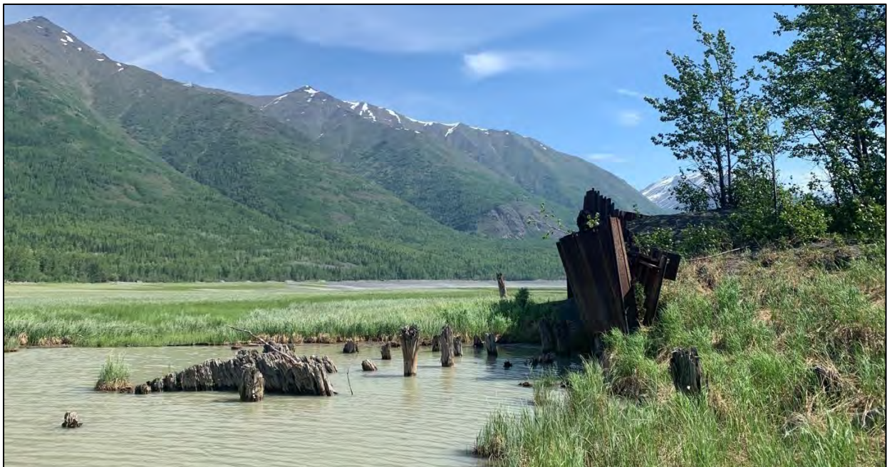
Figure 5.2-8. Feature 2 abutment with an irregular cluster of piers and planks in the center of the lake outlet. View to the northeast.
