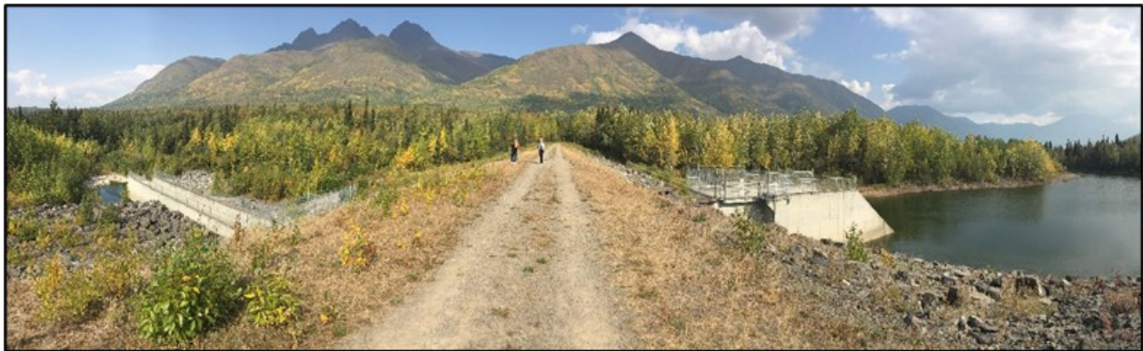
Figure 3-1. Dam Crest and Ungated Overflow Spillway, Looking North.
